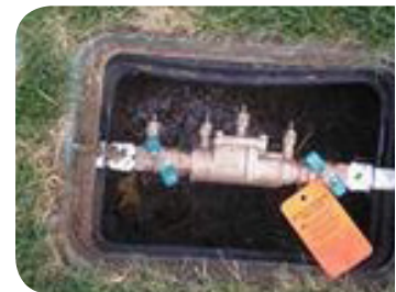
The most common residential backflow device is a DCVA, a double check valve assembly.
