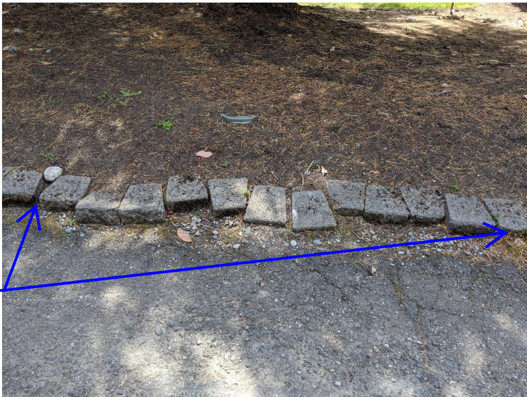
Approximate Station = 440' Looking South.
