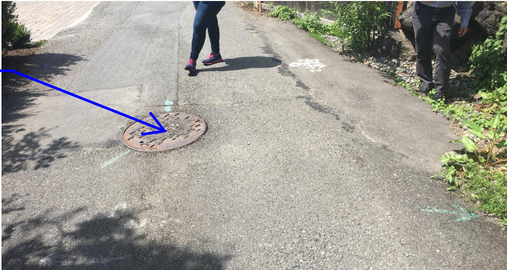
Approximate Station = 390' Looking West.
