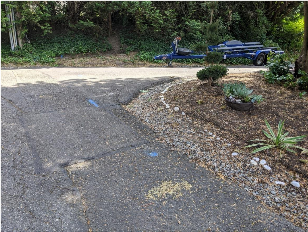
Approximate Station = 550' Looking Southeast.
