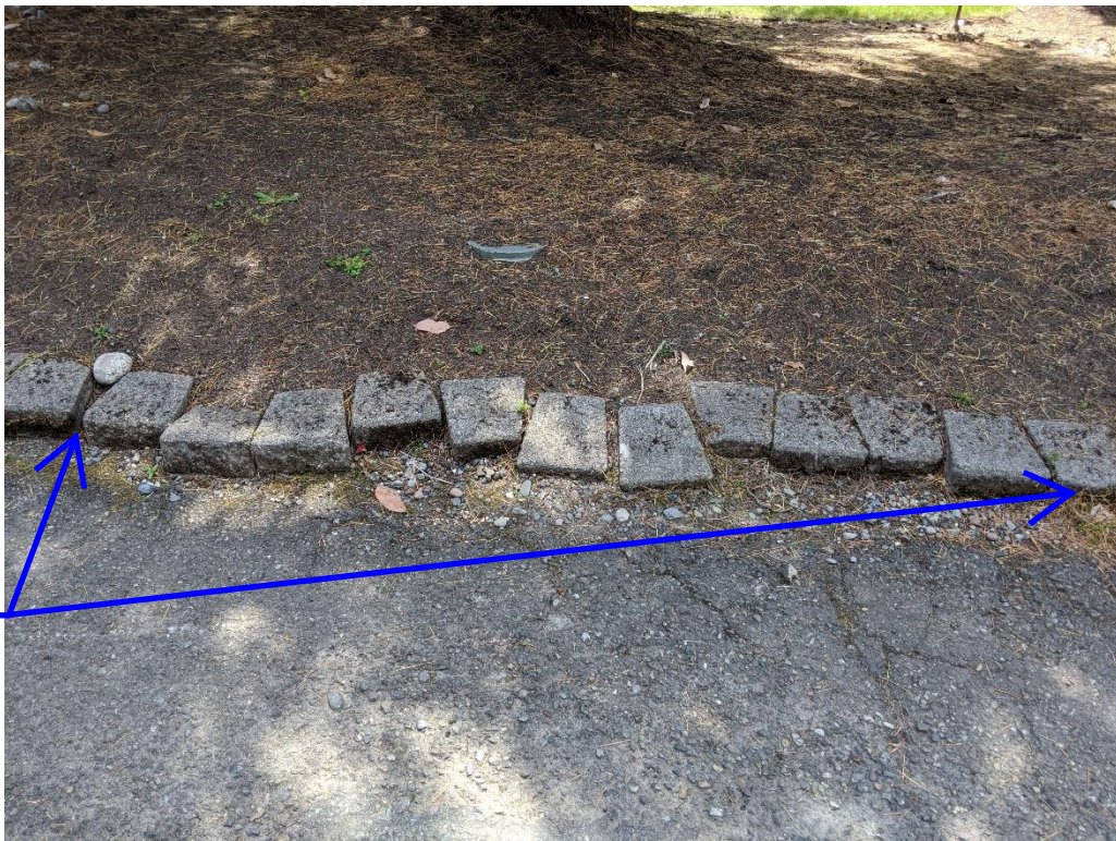
Approximate Station = 440' Looking South.
