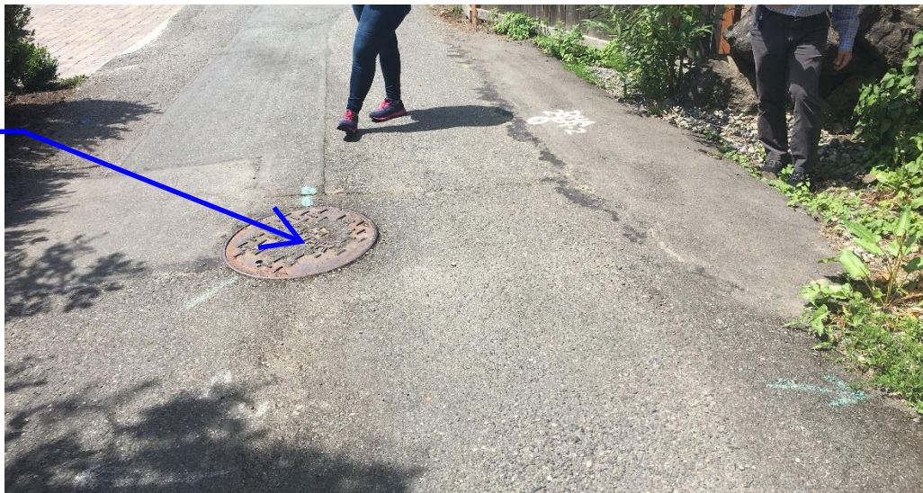
Approximate Station = 390' Looking West.
