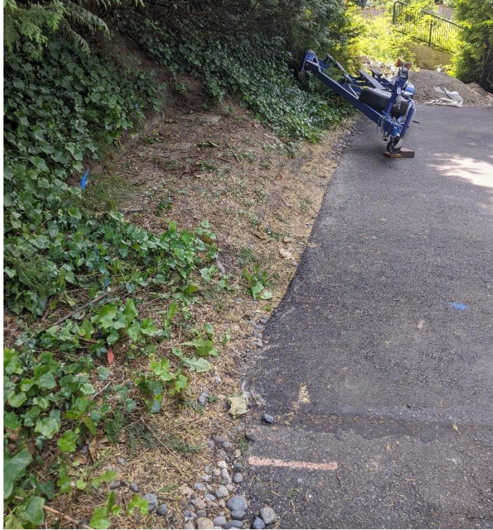
Approximate Station = 570' Looking Southwest at Existing Water Meters.
