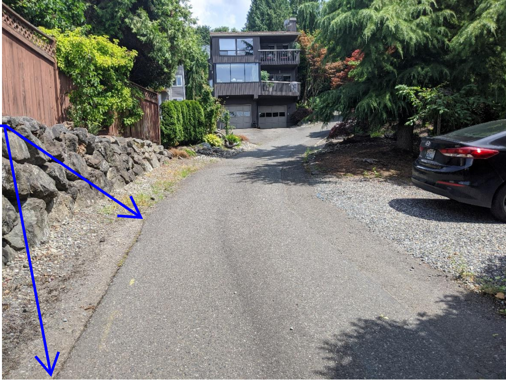
Approximate Station = 395' Looking East
