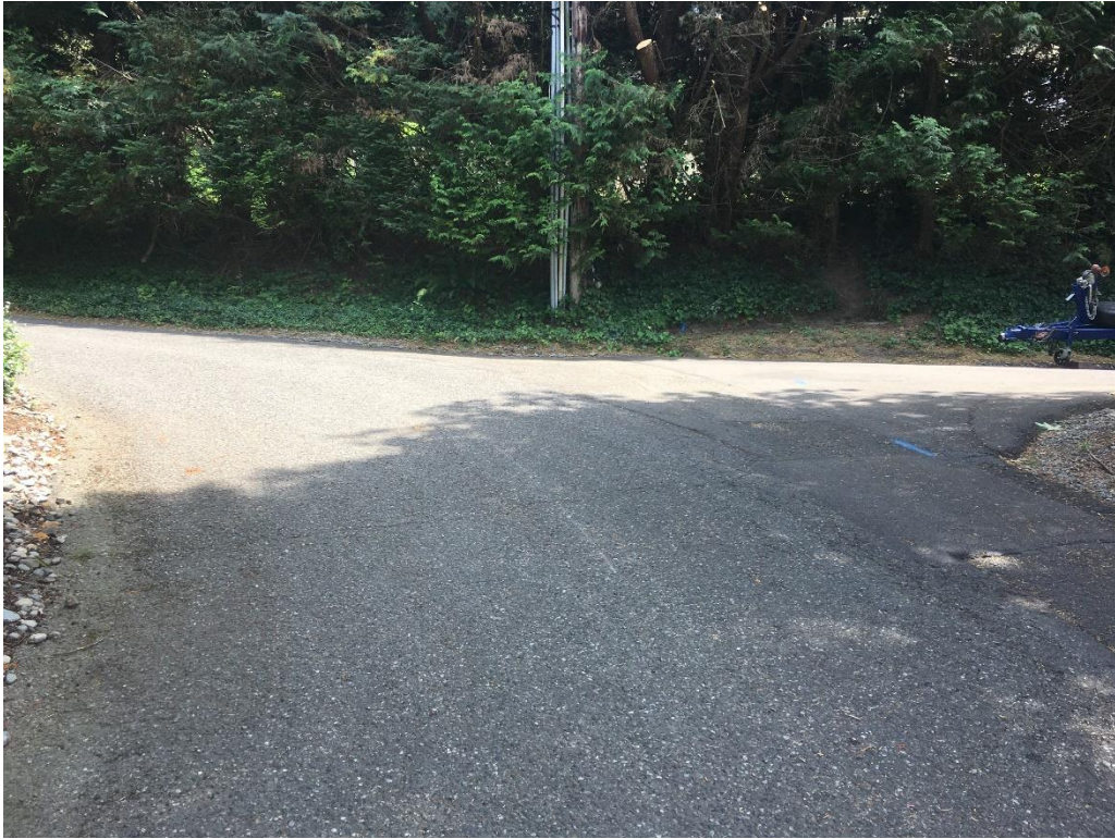
Approximate Station = 545' Looking Southeast.
