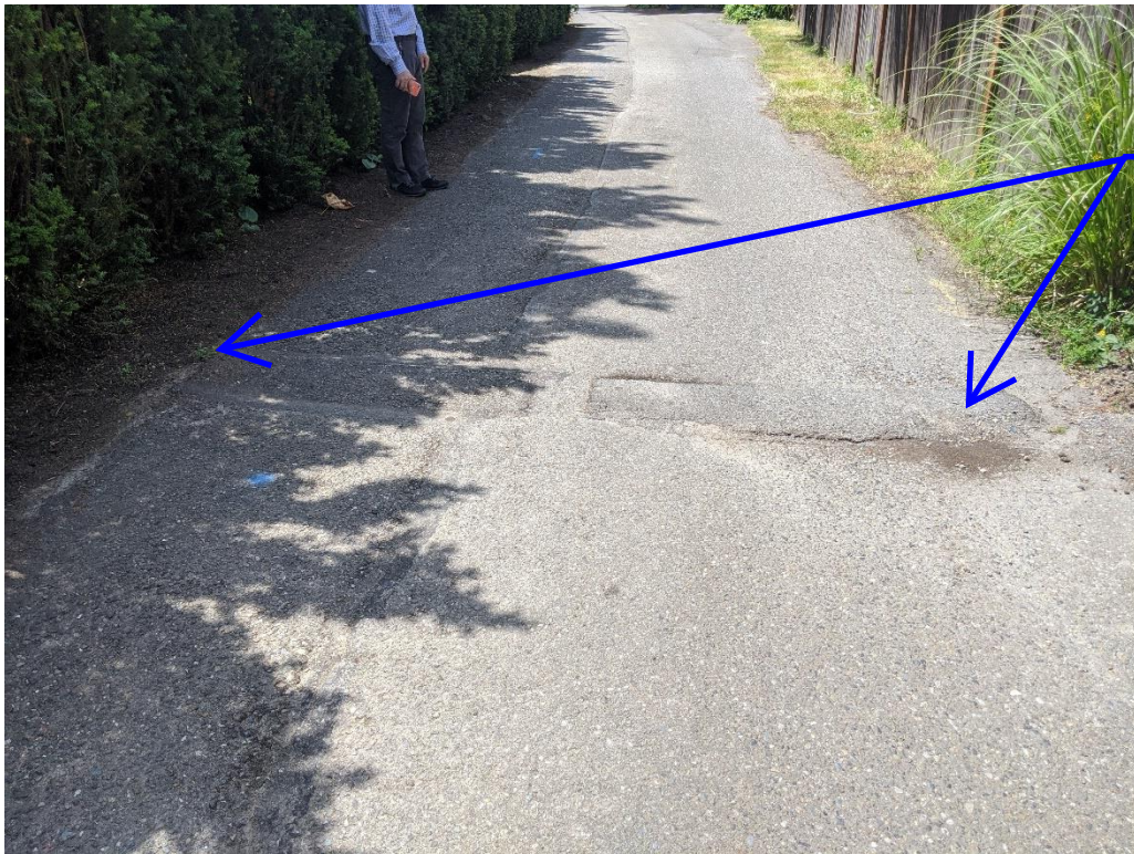
Approximate Station = 285' Looking West.
