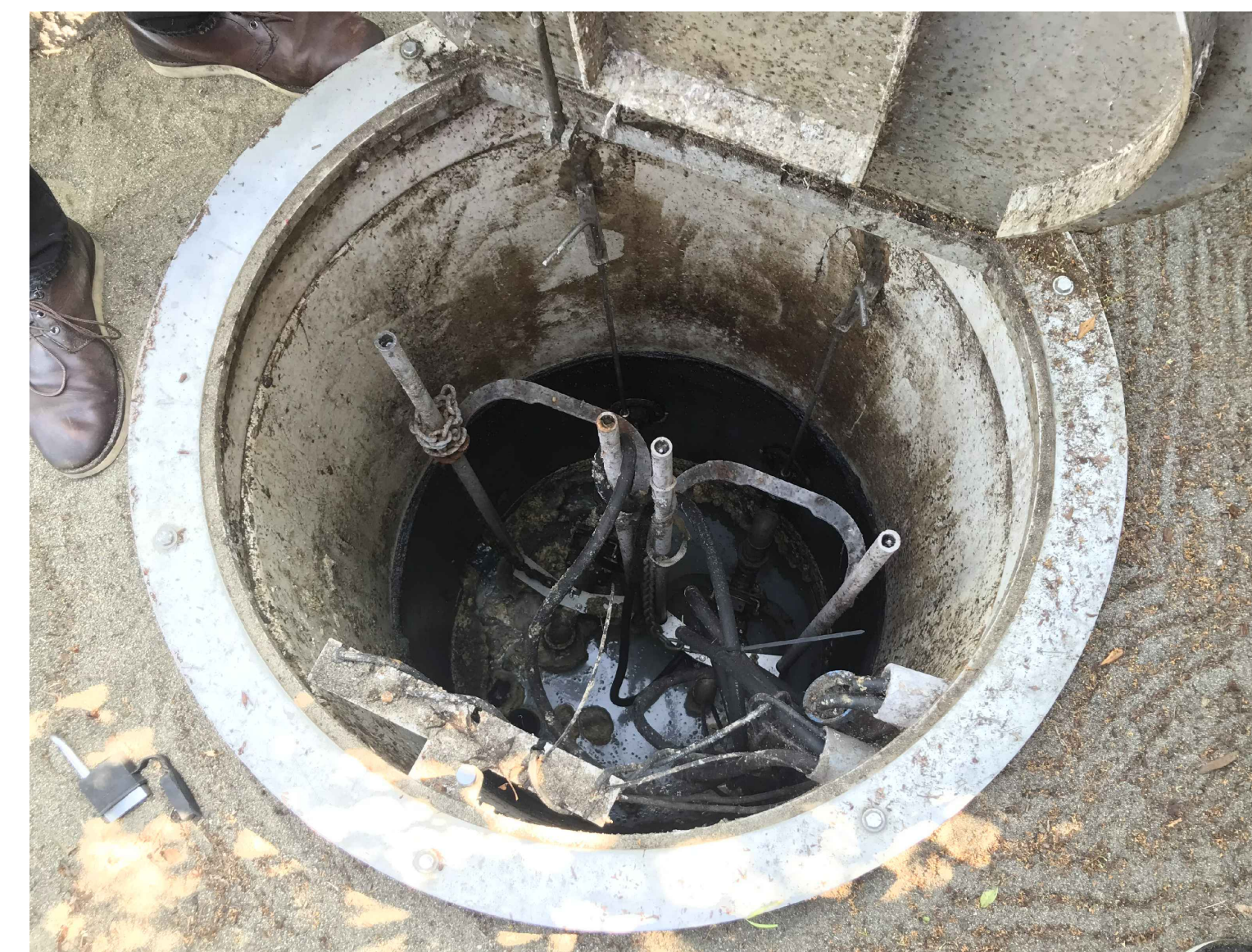
EXISTING WET WELL PHOTOGRAPH
