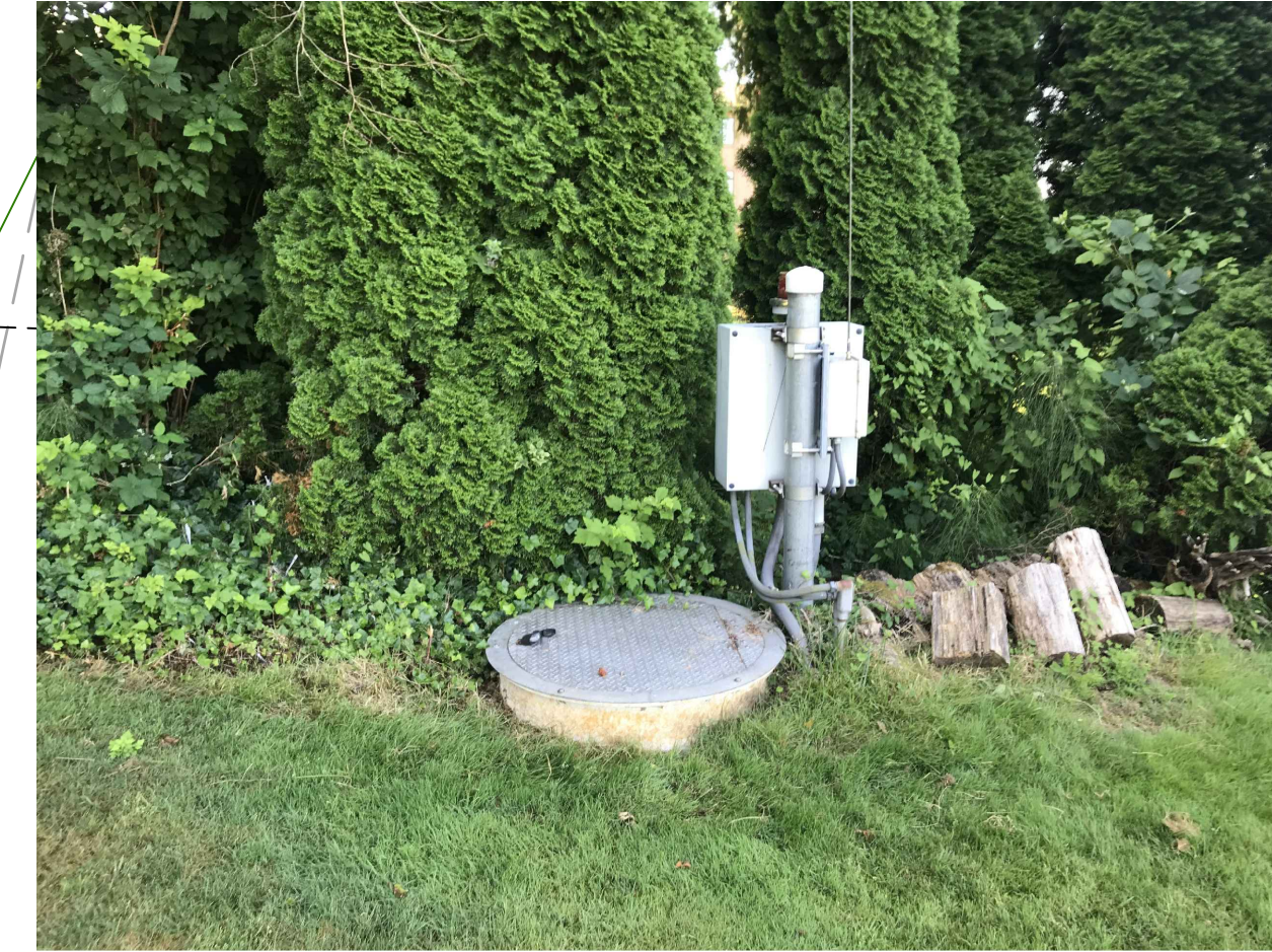
GRINDER PUMP STATION 3 EXISTING SITE PHOTOGRAPH
