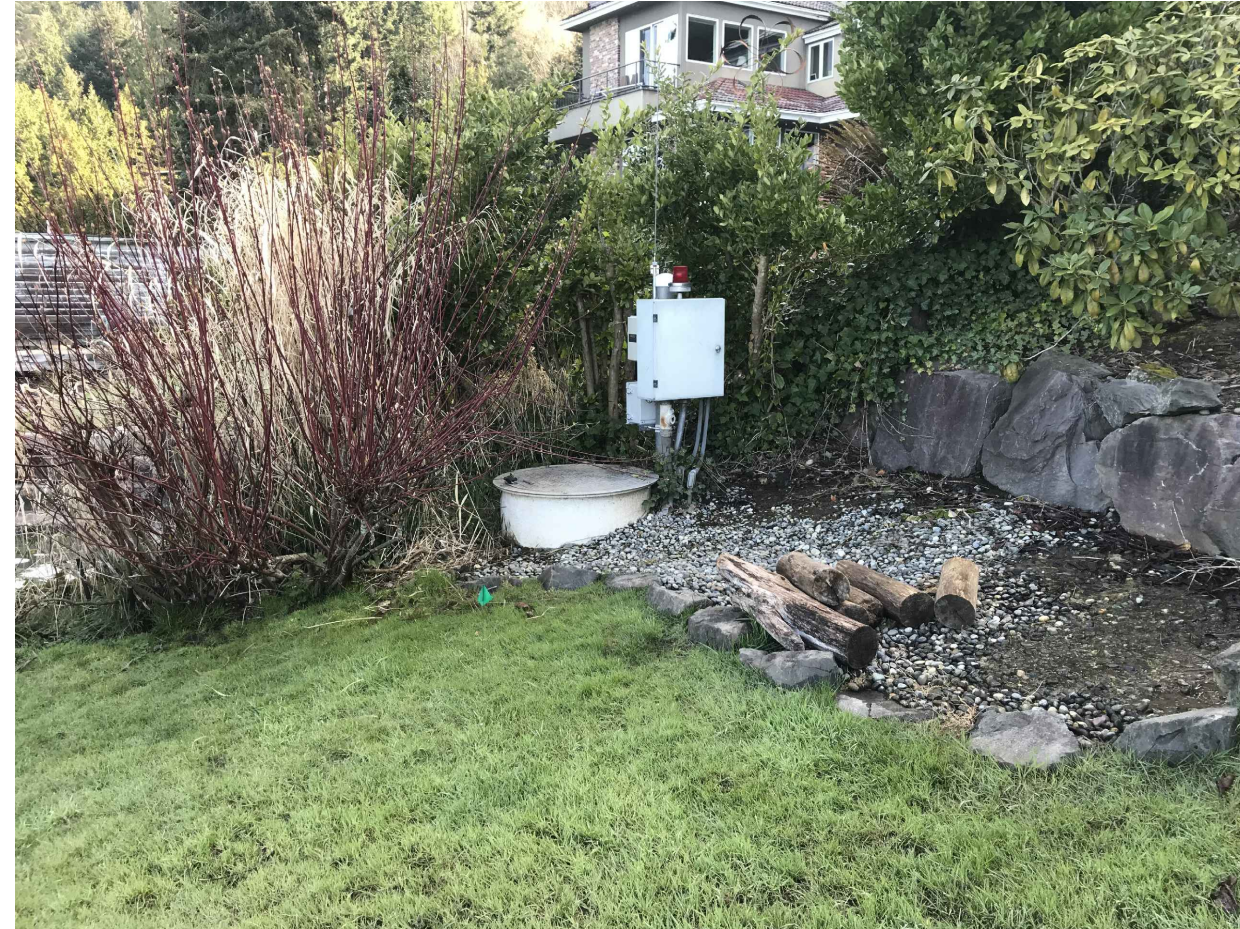
GRINDER PUMP STATION 2 EXISTING SITE PHOTOGRAPH
