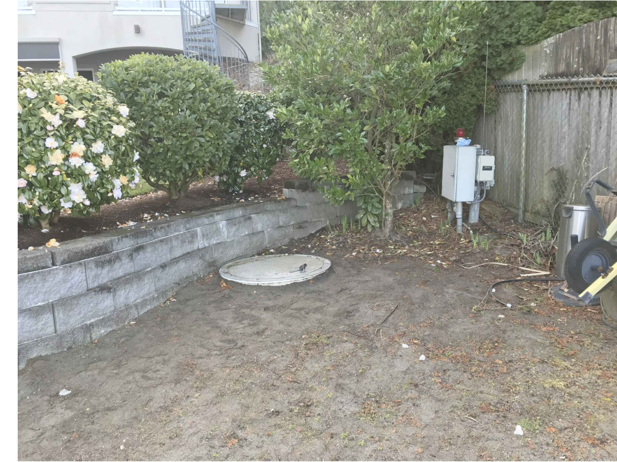
GRINDER PUMP STATION 1 EXISTING SITE PHOTOGRAPH
