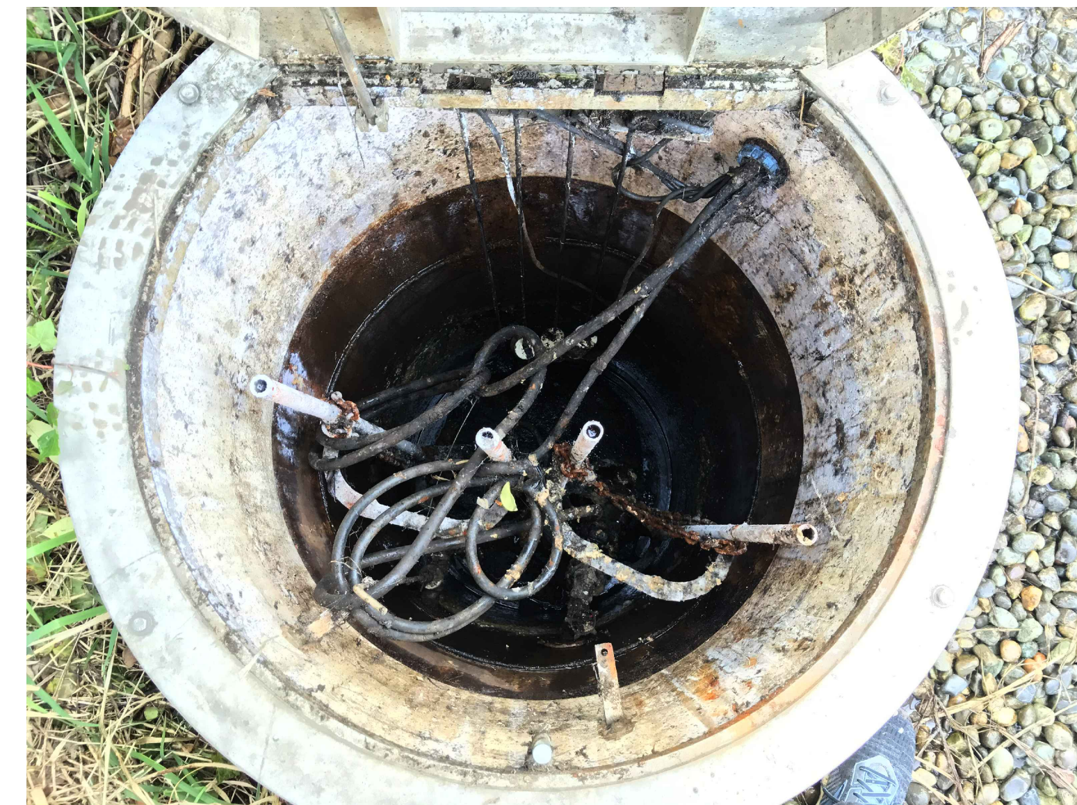
EXISTING WET WELL PHOTOGRAPH
