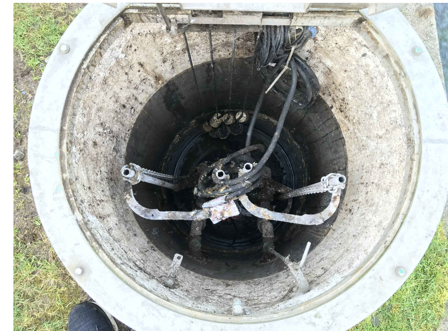
EXISTING WET WELL PHOTOGRAPH
