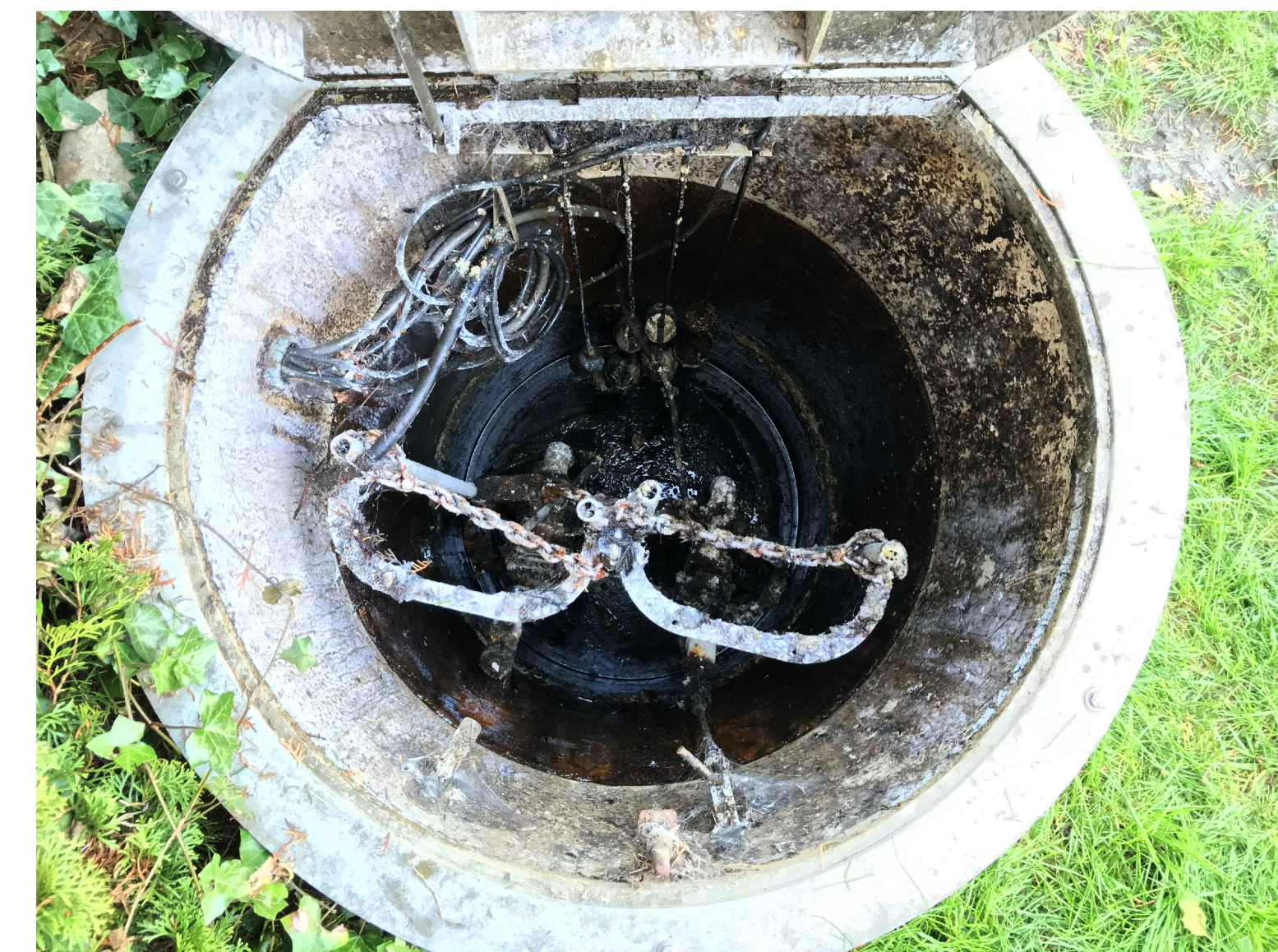
EXISTING WET WELL PHOTOGRAPH
