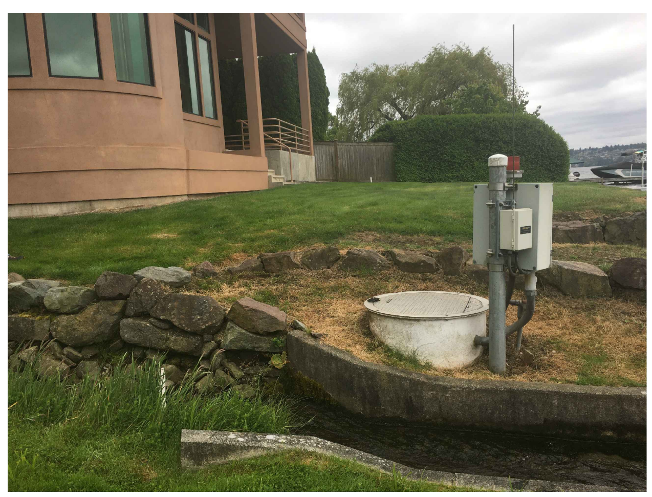
GRINDER PUMP STATION 4 EXISTING SITE PHOTOGRAPH
