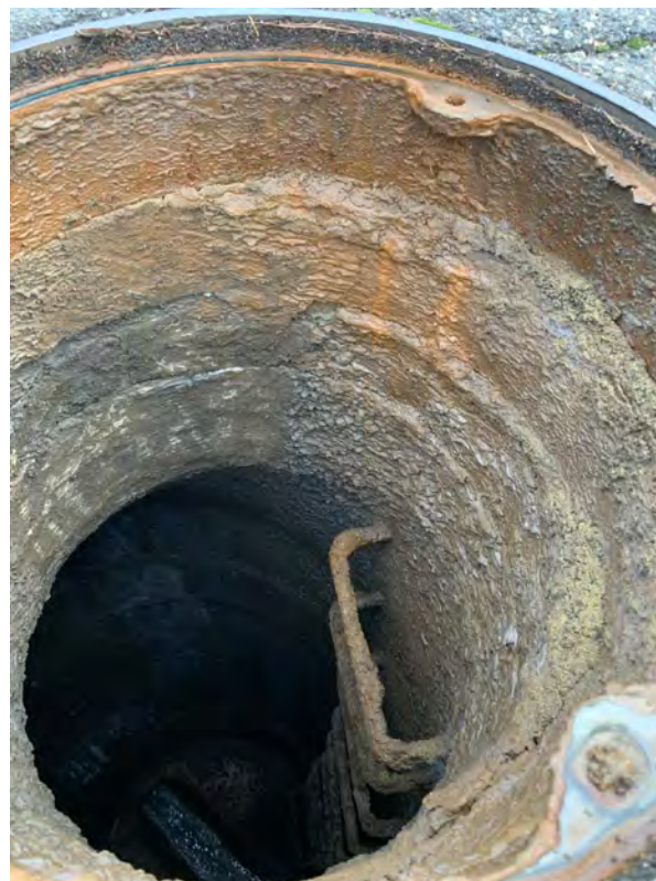
MH - 165 - REPLACE FRAME, COVER AND 10" OF ADJUSTMENT RINGS.
