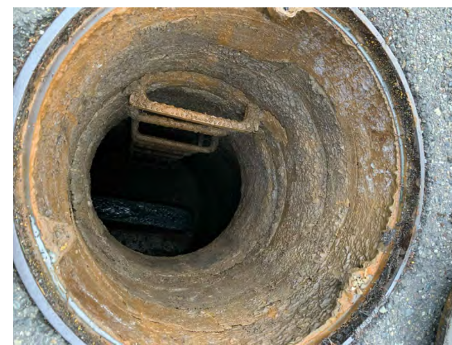
MH - 161 - REPLACE FRAME, COVER AND 18" OF ADJUSTMENT RINGS.
