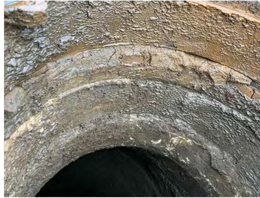
MH - 162 - REPLACE FRAME, COVER AND 10" OF ADJUSTMENT RINGS. PROTECT SURVEY MONUMENT
