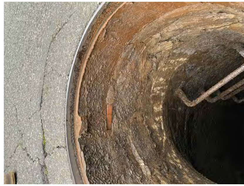
MH - 156A - REPLACE FRAME, COVER AND 10" OF ADJUSTMENT RINGS.
