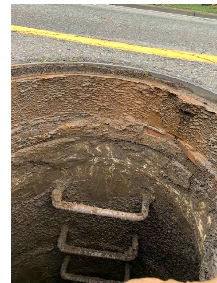
MH - 157 - REPLACE FRAME, COVER AND 8" OF ADJUSTMENT RINGS.
