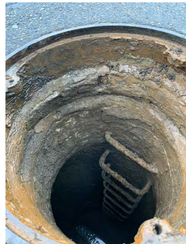
MH - 166A - ADD MAHOLE SECTION, REPLACE MANHOLE CONE, FRAME, COVER AND ADJUSTMENT RINGS AS PER DETAIL 3 SHEET 17. CONFIRM KEY-WAY PRIOR TO INSTALLATION. PROTECT SURVEY MONUMENT
