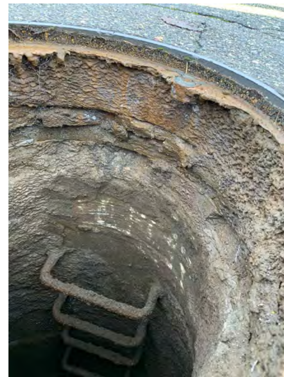
MH - 156 - REPLACE FRAME, COVER AND 18" OF ADJUSTMENT RINGS.
