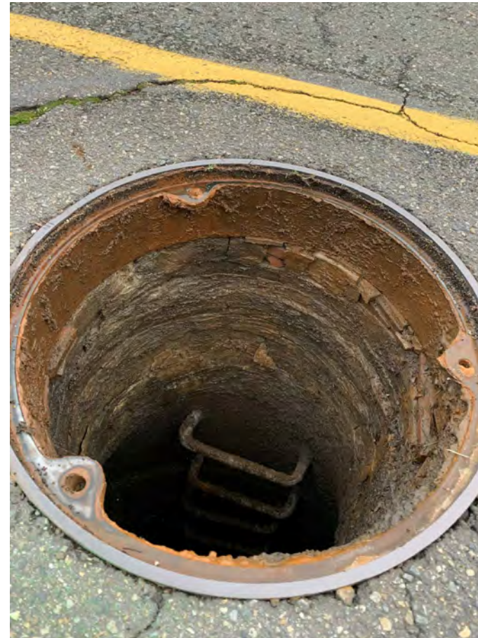
MH - 160 - REPLACE FRAME, COVER AND 18" OF ADJUSTMENT RINGS.
