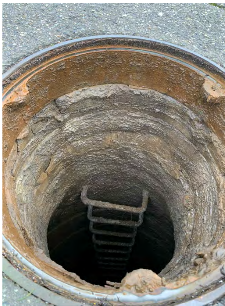
MH - 159 - REPLACE FRAME, COVER AND 18" OF ADJUSTMENT RINGS.
