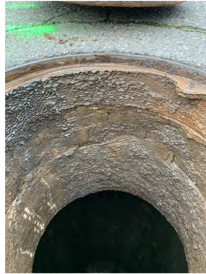
MH - 166 - REPLACE FRAME, COVER AND 8" OF ADJUSTMENT RINGS.
