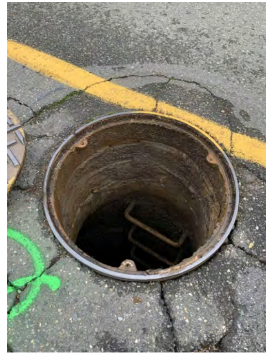
MH - H722 - REPLACE FRAME, COVER AND 10" OF ADJUSTMENT RINGS.
